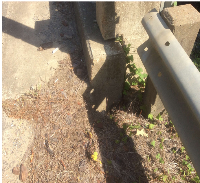
PHOTO 1 Description Bent 3 south east bridge end small area of erosion at end post.
